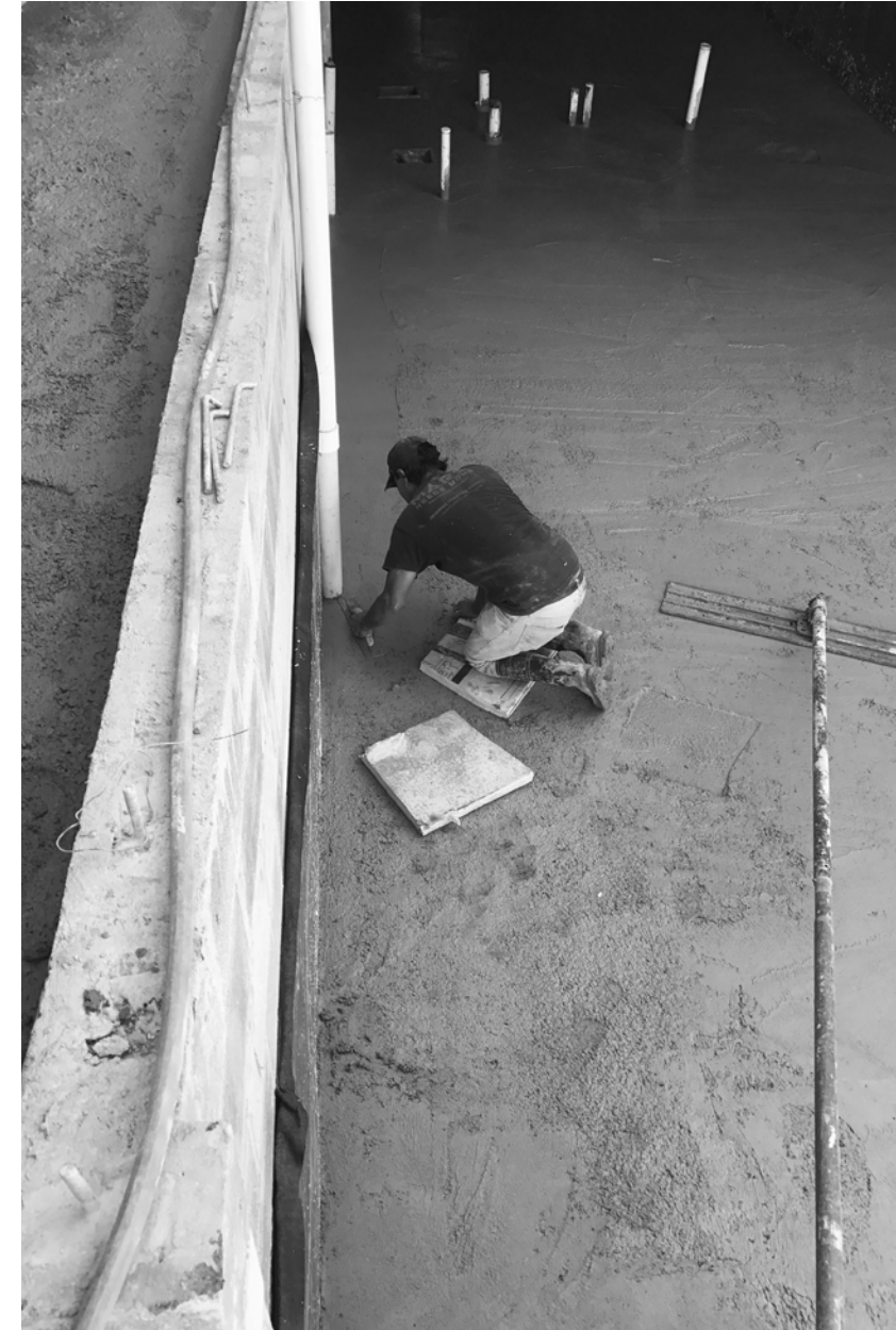
A construction worker carefully smooths and buffs the concrete slab, which was one of the most technically challenging parts of the project.
