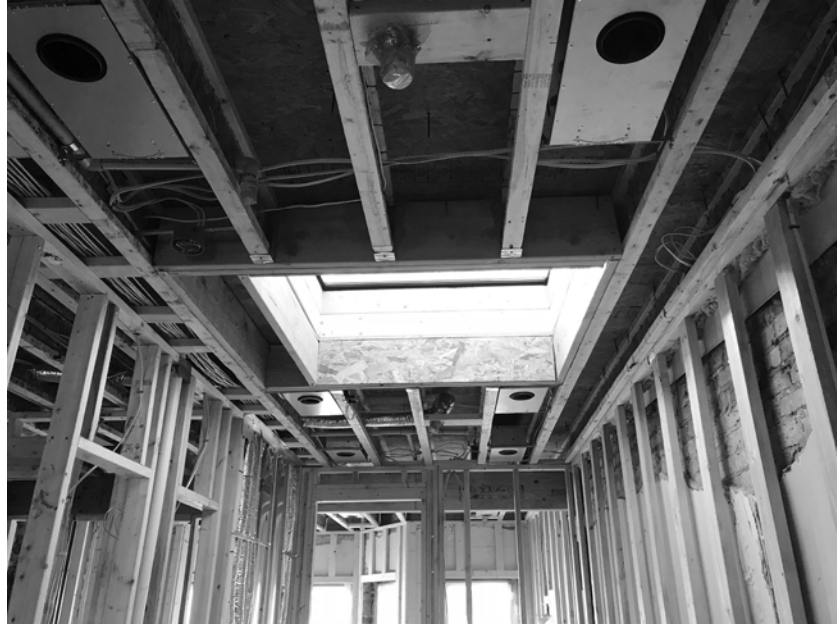
Integrated LED lights and a skylight were installed after deconstruction of the old roof.
