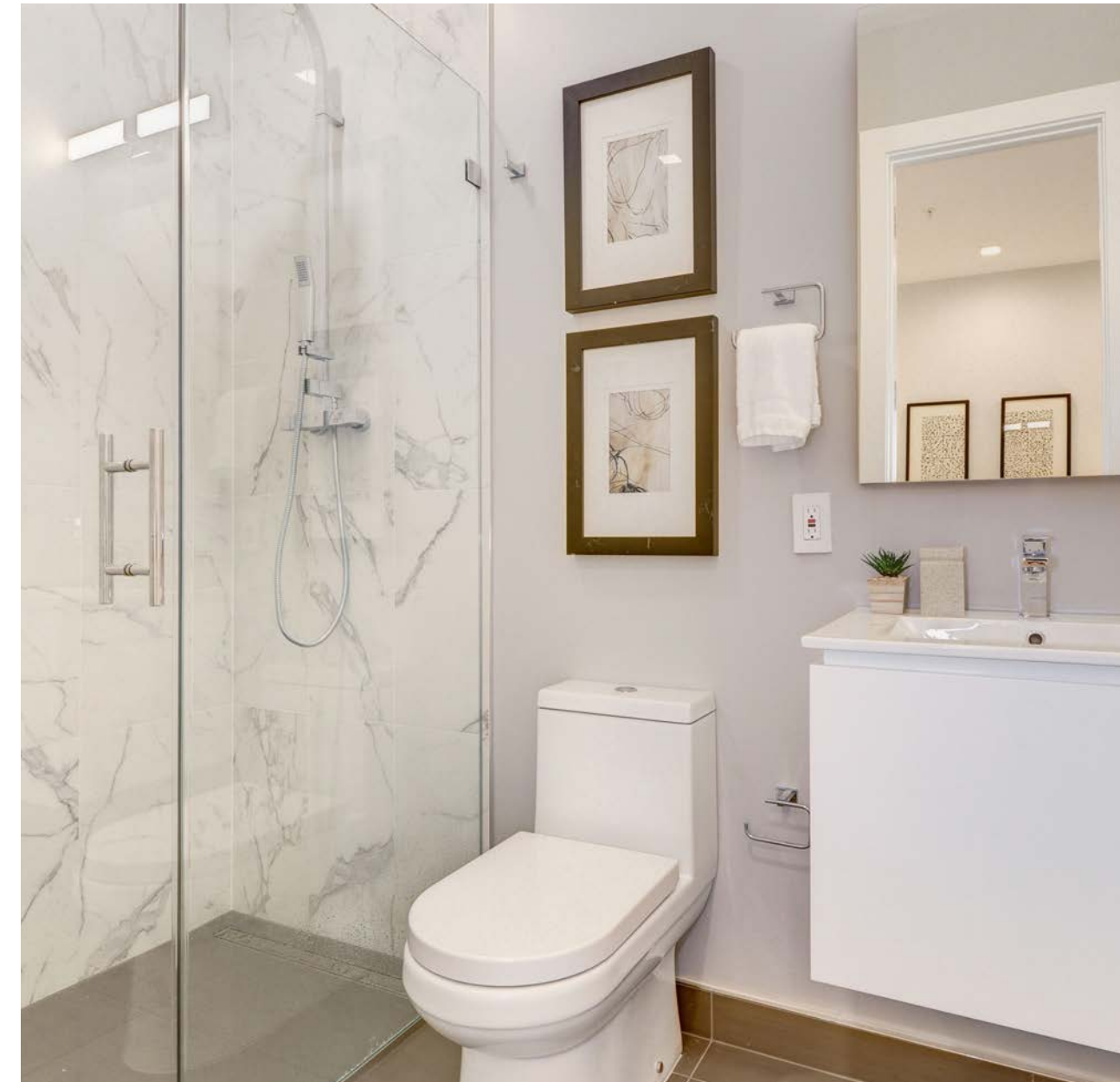
The bathrooms feature oversized porcelain wall tiles, efficient flush toilets, and curbless shower floors with linear drain systems.
