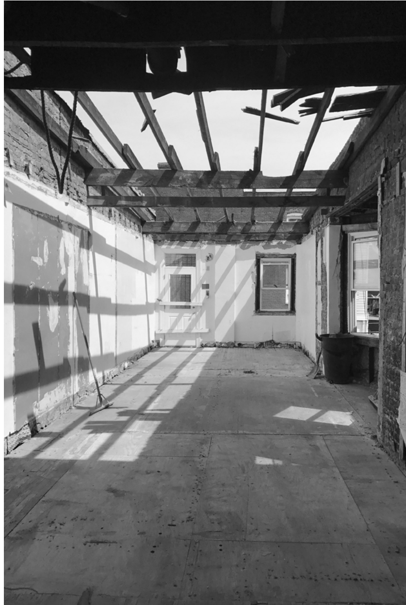
Integrated LED lights and a skylight were installed after deconstruction of the old roof.
