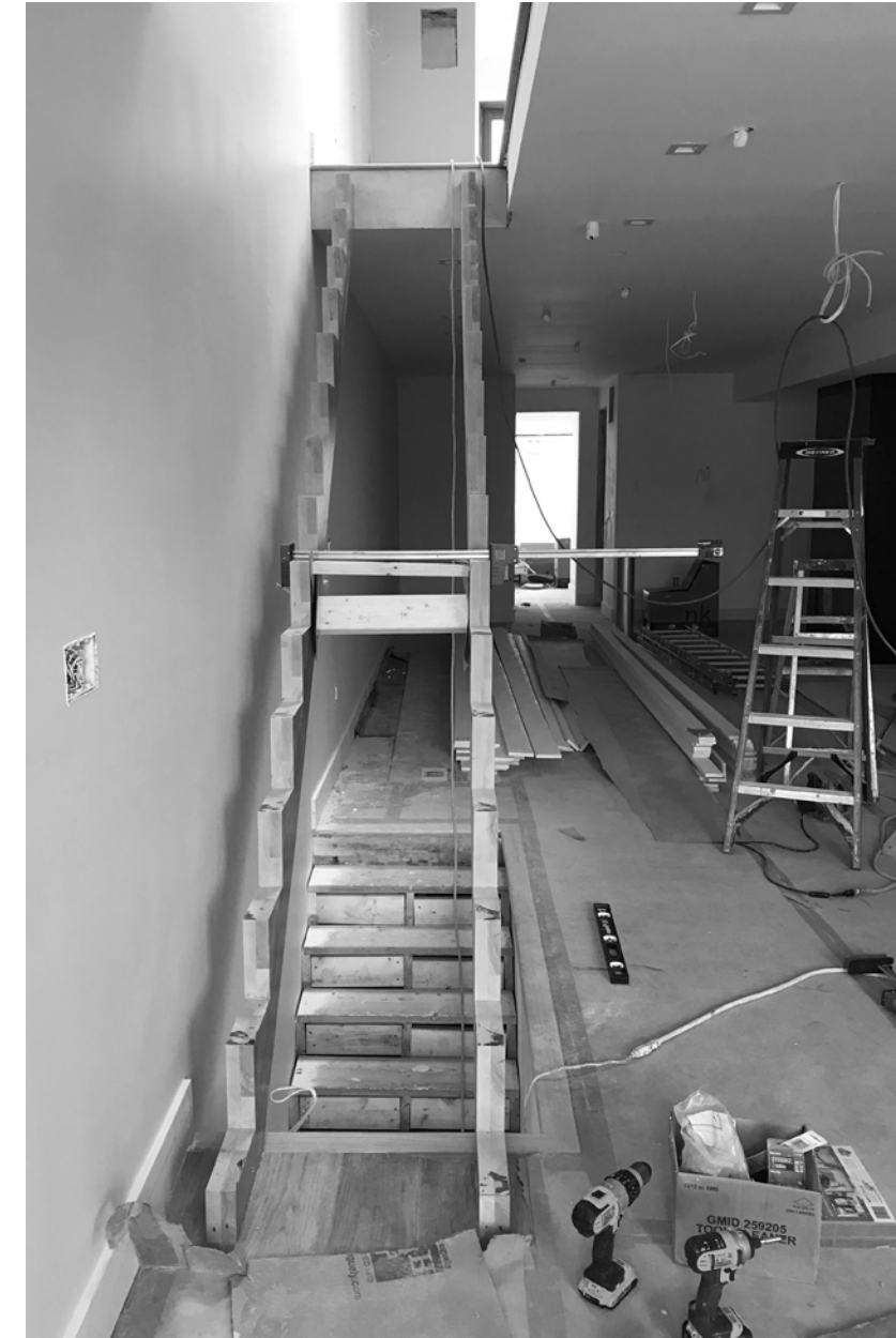
The new staircase was constructed with Ashwood and features an open riser and sleek glass design.
